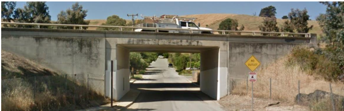
Figure 1 Washington Street Underpass North Façade (View Looking South)
