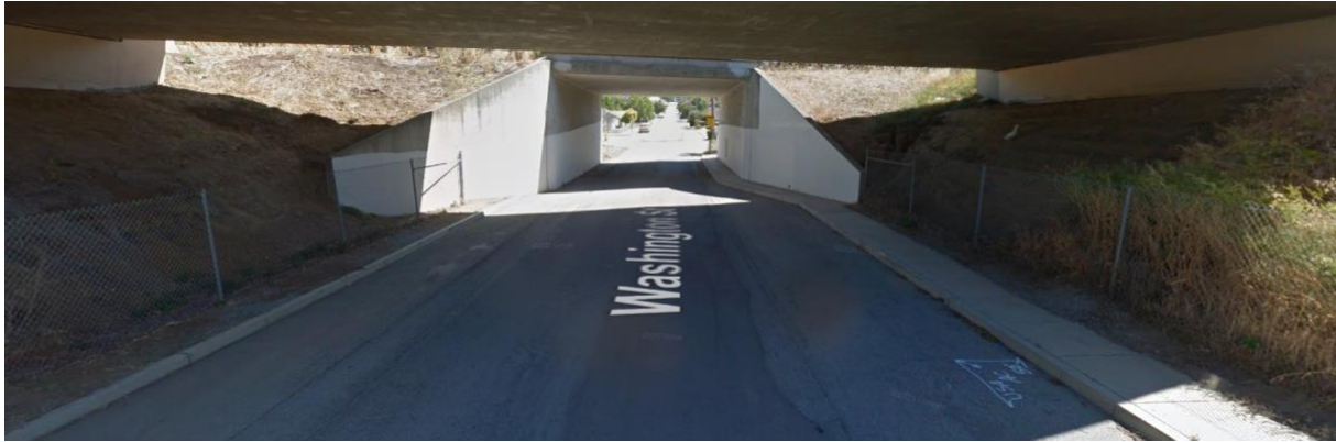
Figure 3 Washington St Underpass Inside Walls and South Façade (View Looking North)
