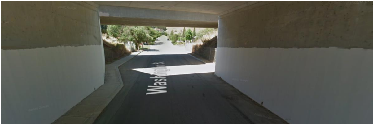
Figure 2 Washington St Underpass Inside Walls (View Looking South)
