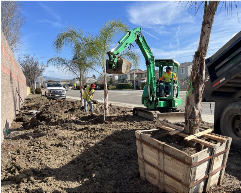
Landscape construction in progress Spring 2024
